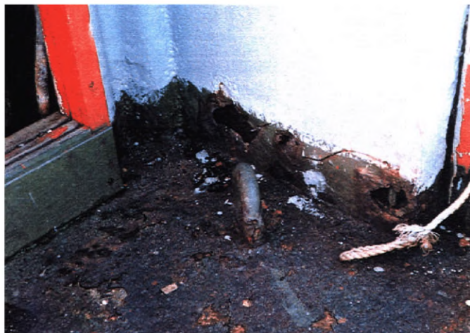
Photograph 1 Corroded accommodation house side structure
