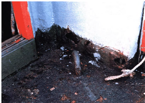
Photograph 1 Corroded accommodation house structure
