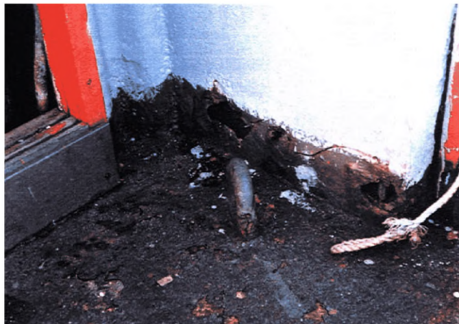
Photograph 1 Corroded accommodation house side structure
