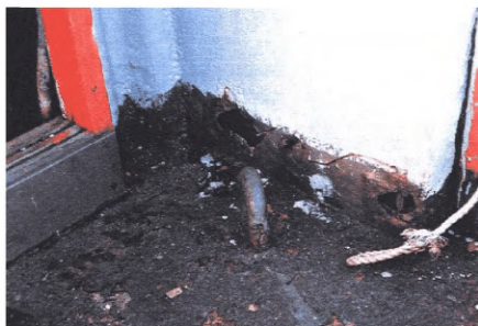
Photograph 1 Corroded accommodation house side structure
