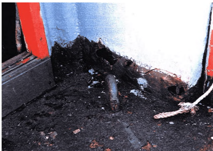
Photograph 1 Corroded accommodation house structure
