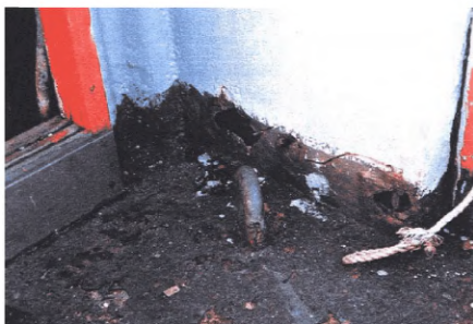
Photograph 1 Corroded accommodation house side structure
